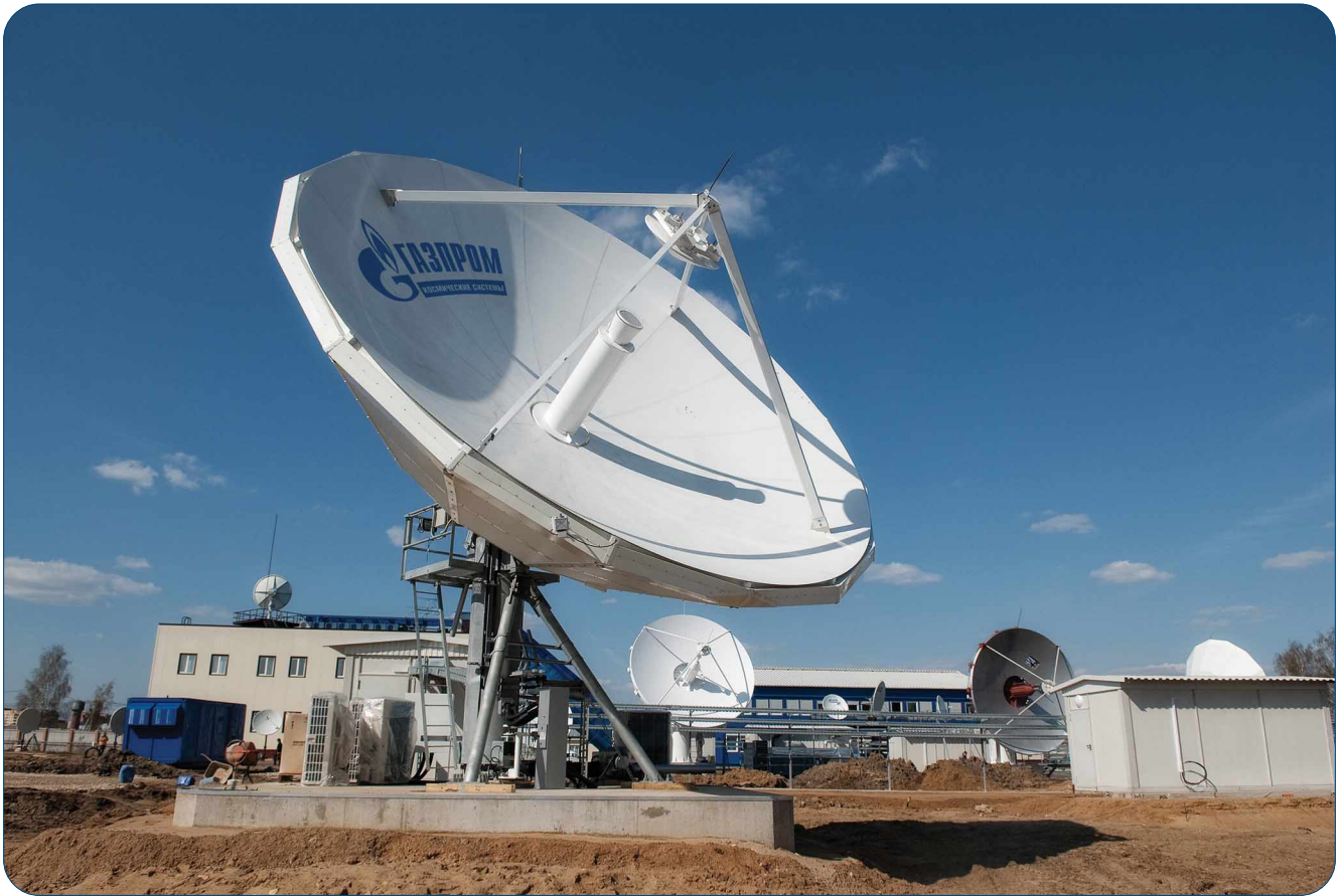
New GSS Telecommunication Centre.
