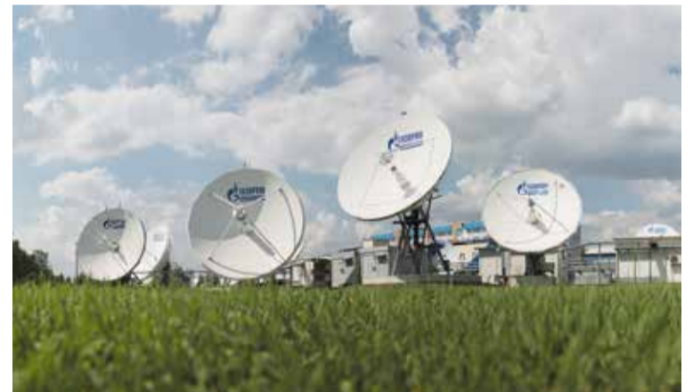
Gazprom Space Systems Telecommunication center
